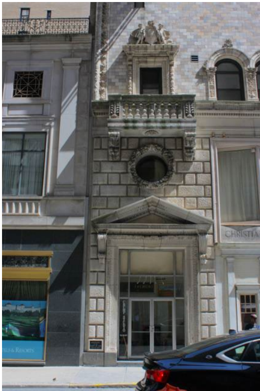
Figure 5. Façade (west elevation): Left (north) entrance.
