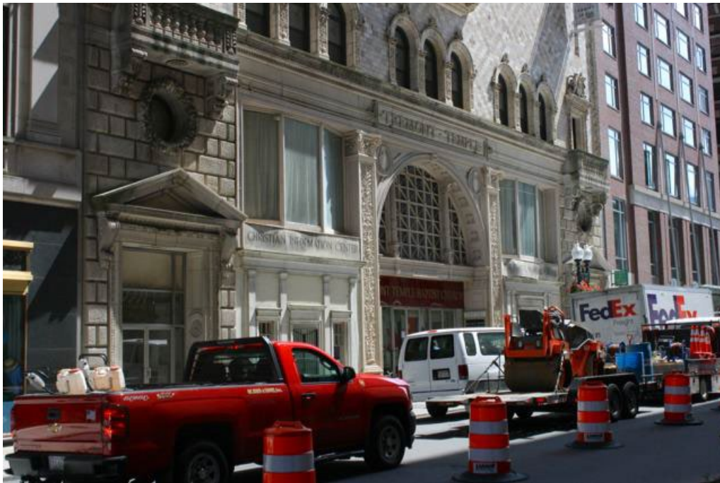
Figure 3. Façade (west) elevation: Base of building with storefronts and entrances.
